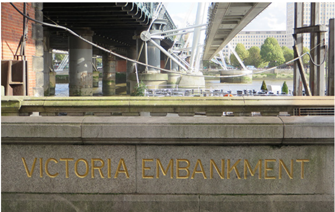
Victoria Embankment, underneath Hungerford Bridge.
